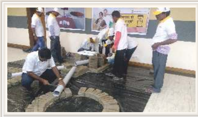
Twin Pit Toilet Technology workshop for Masons in Odisha in July
